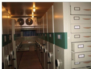
Cold room (-5 °C)
